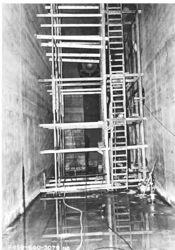
B. Installation of transducers in outlet stilling basin wall.
