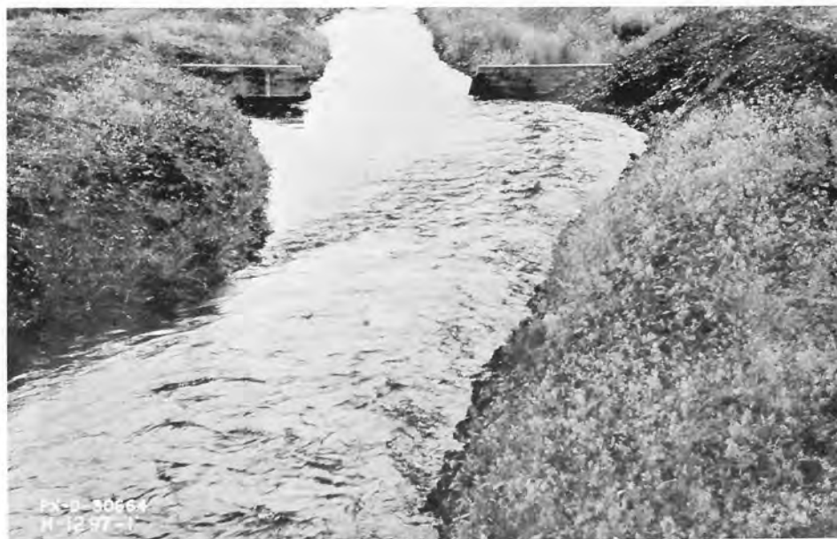
Poor approach flow conditions upstream from weir. The high-velocity, turbulent stream is approaching the weir at a considerable angle. Head measurement is difficult, and weir does not discharge a "standard" quantity. PX-D-30664
