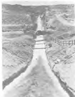
FIG. 1.—AIR ENTRAINMENT FROM SIDE-GENERATED TURBULENCE
