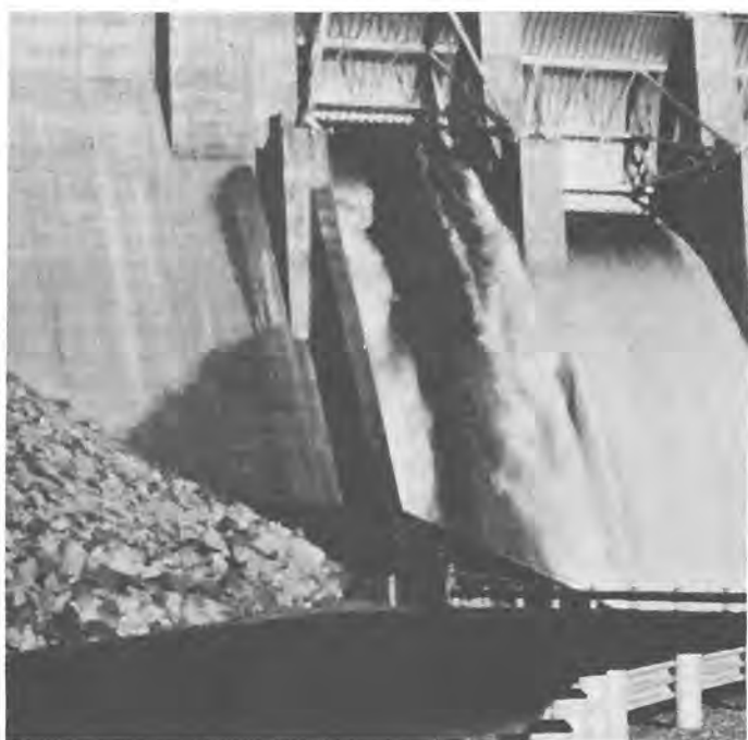
FIG. 5.—EFFECT OF SPILLWAY PIERS ON AIR ENTRAINMENT
