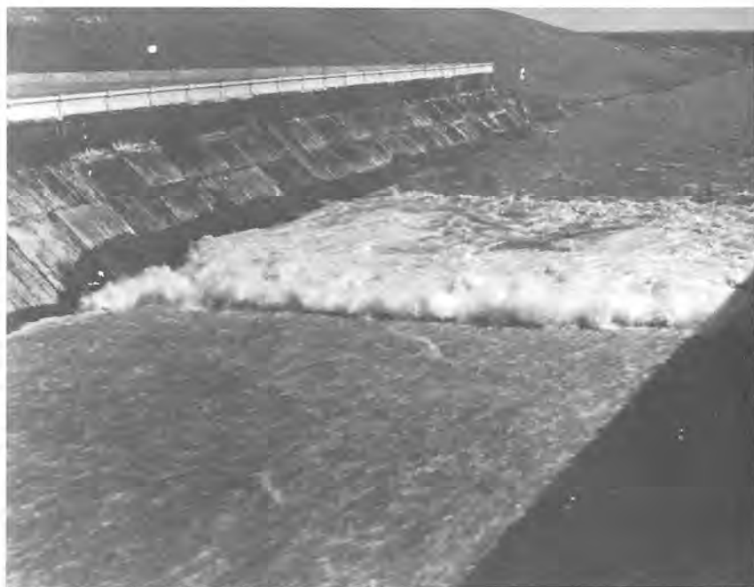
FIG. 3.—LOW AIR ENTRAINMENT FROM BOTTOM-GENERATED TURBULENCE IN A WIDE SPILLWAY CHUTE
