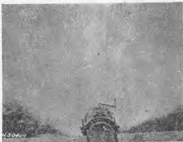
Fig. 6a — 6-inch valve discharging with hood removed
