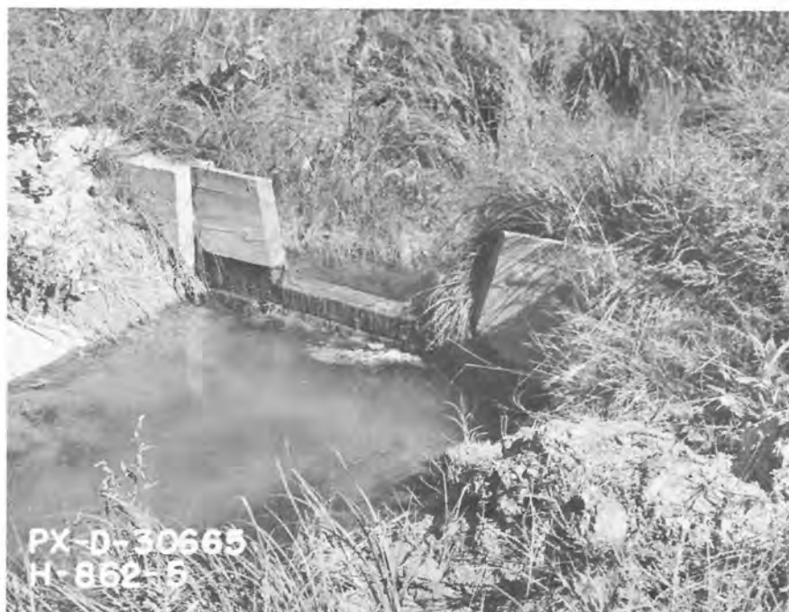
Weeds protruding through the opening and sediment in the approach pool will result in inaccurate discharge determinations. PX-D-30665 Figure 9
