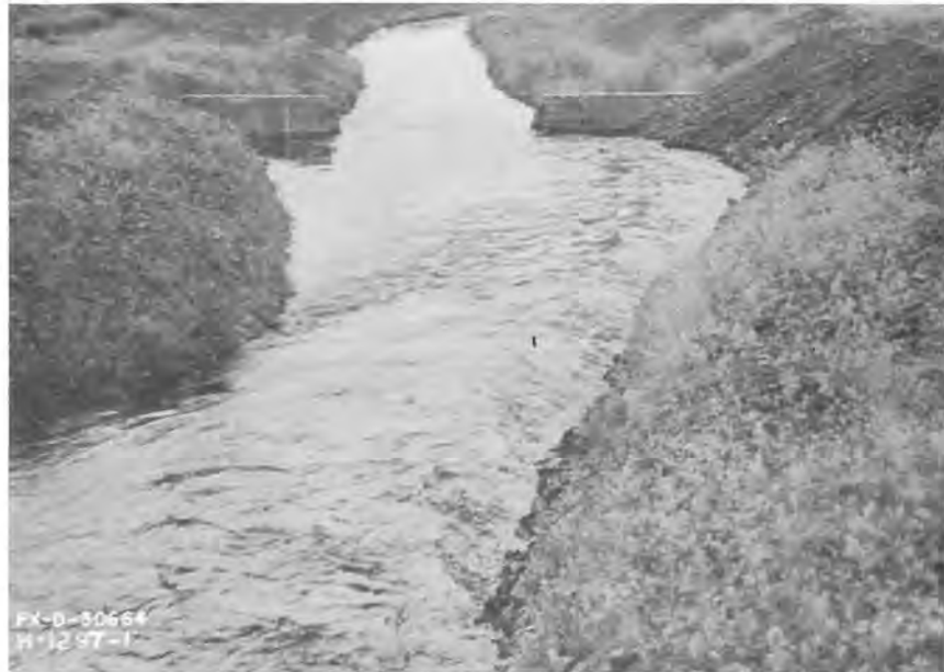
Poor approach flow conditions upstream from weir. The high-velocity, turbulent stream is approaching the weir at a considerable angle. Head measurement is difficult, and weir does not discharge a "standard" quantity. PX-D-30664 Figure 1
