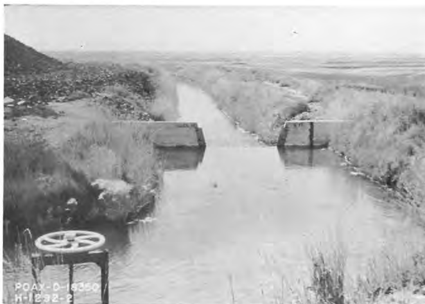
Cippoletti weir operating with good flow conditions in the approach pool. Flow is well distributed across wide pool and shows no evidence of excessive turbulence. Accurate or "standard" discharges can be expected under these conditions.
