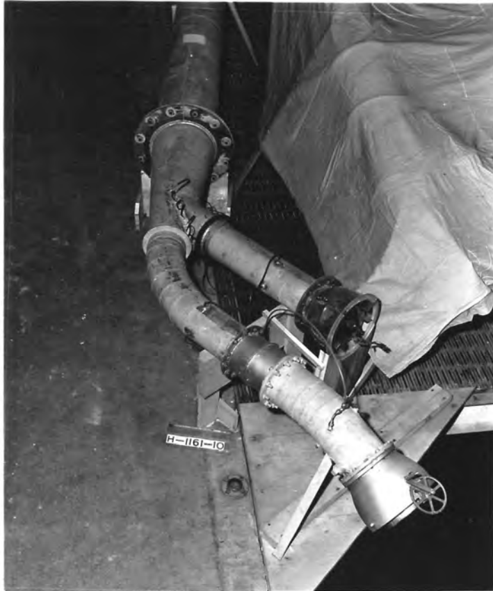
Figure 1, 1:15 Scale Model, Outlet Works, Mexican Side, Falcon Dam.
