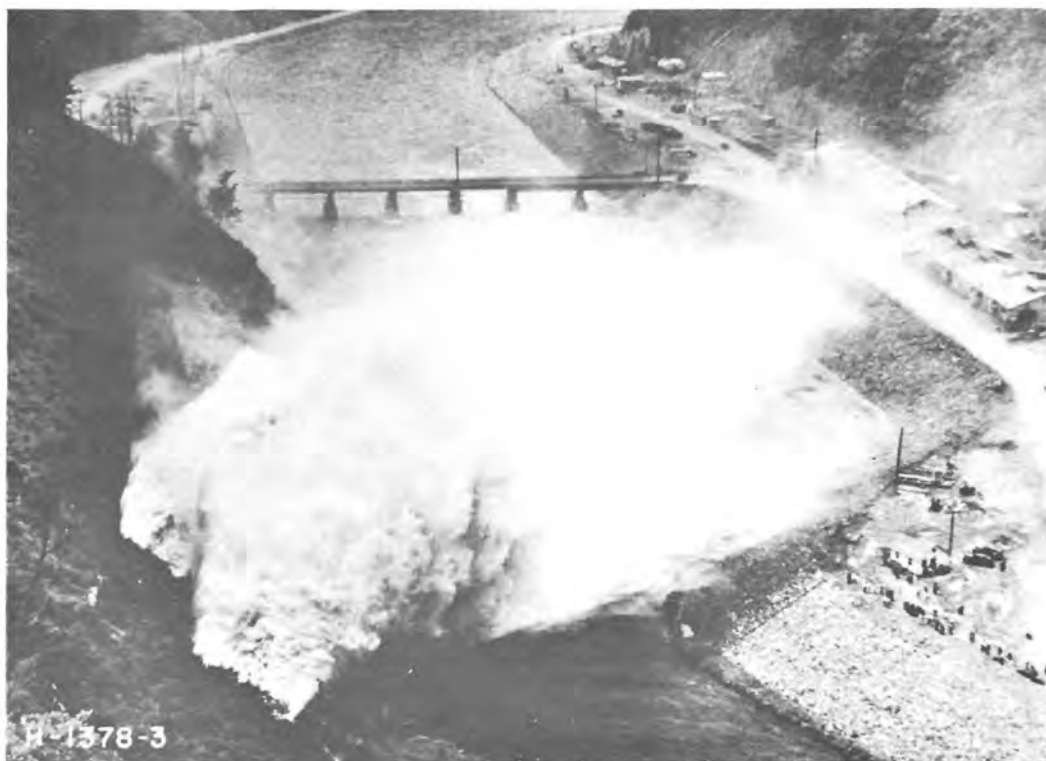
Both Prototype Tunnels discharging 10,000 cfs each. P-232-D-17059
