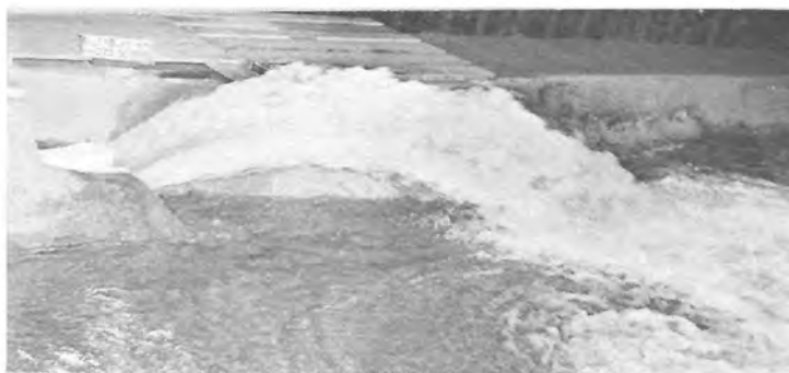
TYPICAL JET PROFILE 35° TRANSITION FLIP BUCKET P-557-D-17053
