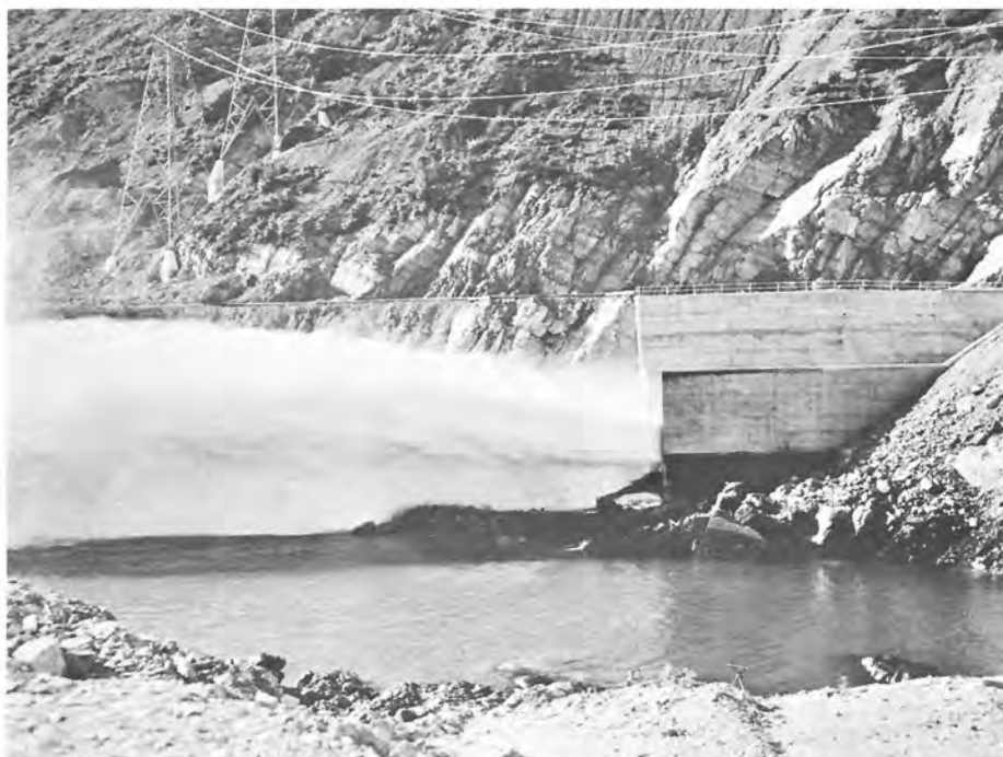
HH-5921 - Hungry Horse spillway tests. Spillway discharge 30,000 c.f.s. Side view of jet under cables. 5:30 p.m. 7-13-54
