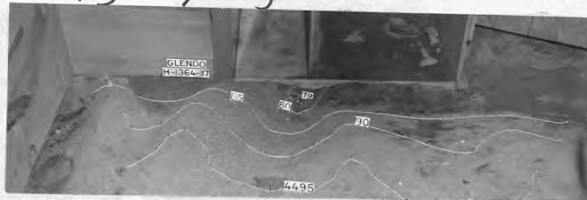
B. Erosion in d.s. channel after 1-hour operation at 83% gate opening. Q=10,000 cfs. N.T.W. + 1\frac{1}{2} feet.
