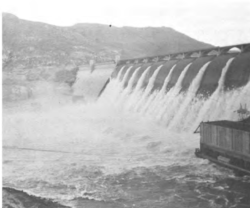
Spillway of Grand Coulee Dam releasing about 500,000 cfs; about 50 percent of design capacity. (H-740-30)
