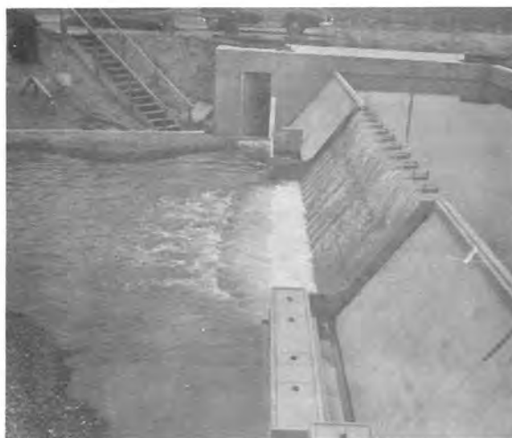
1 to 60 scale model of Grand Coulee Dam, Spillway and Powerplants used mainly to study flow conditions as related to protection of downstream river banks and channel. Spillway releasing flow representing 500,000 cfs or 50 percent of capacity. Model is located on the shore of Lake Roosevelt upstream from the left abutment of the dam. (H-843-181)
