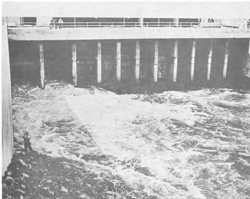
Figure 37. Flow Conditions in Tailrace Downstream of Boysen Dam Outlet Works Stilling Basin--About 1,400 cfs.
