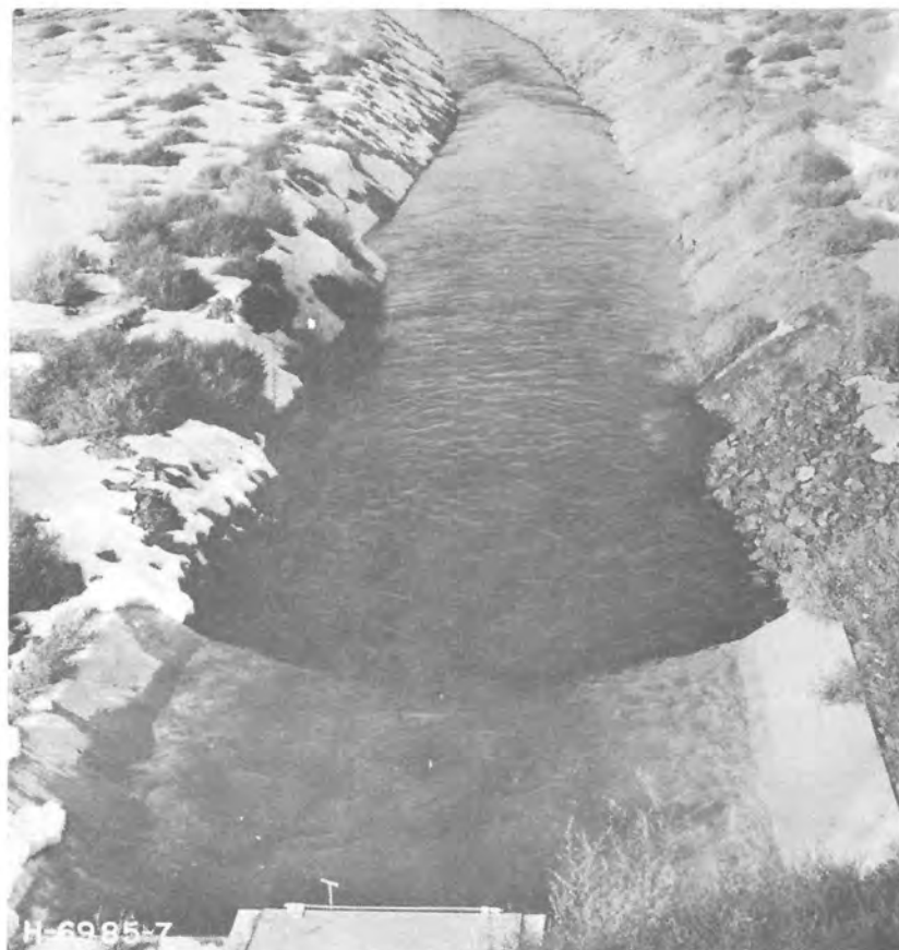
Figure 29. Soap Lake Siphon Blowoff Stilling Well Discharging About 85 cfs. Under 150-foot Head.
