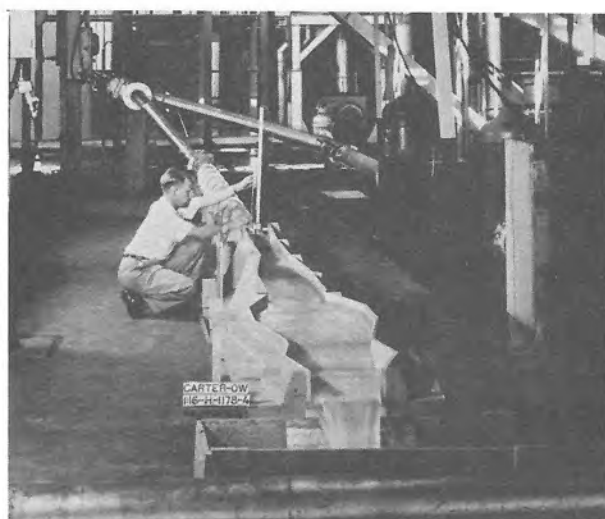
Figure 4. Model of Carter Lake Outlet Works--Scale 1 to 16.
