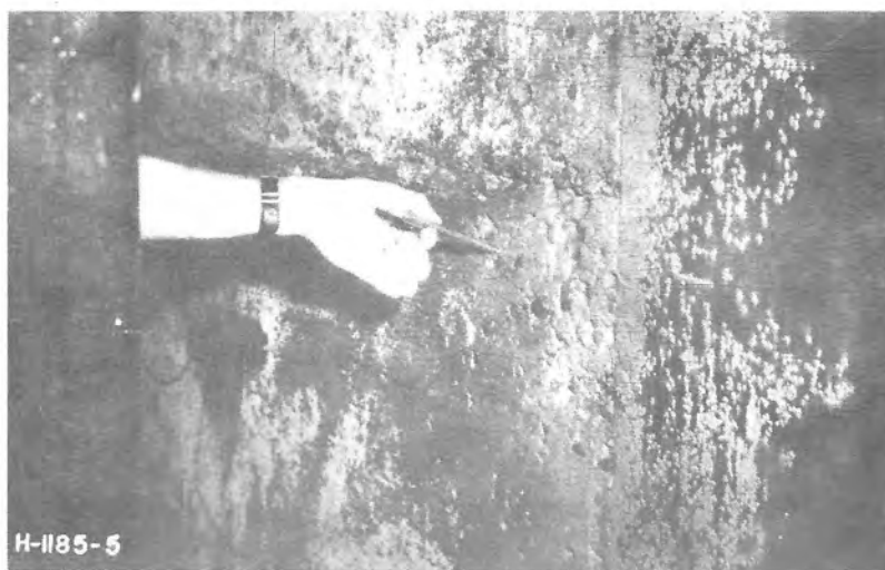
Figure 23. Flatiron Power and Pumping Plant--Cavitation at Into-the-Flow Offset of Concrete Wall in Stilling Basin.
