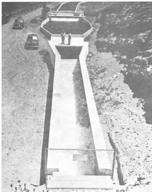
Figure 10. Carter Lake Outlet Works Stilling Basin and Parshall Flume--Modified Structure--Jump Stays in Stilling Basin--380 cfs.
