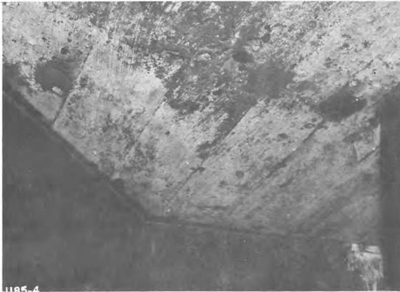
Figure 24. Flatiron Power and Pumping Plant-- Cavitation in Coiling of Stilling Basin Downstream of Triangular Baffle.
