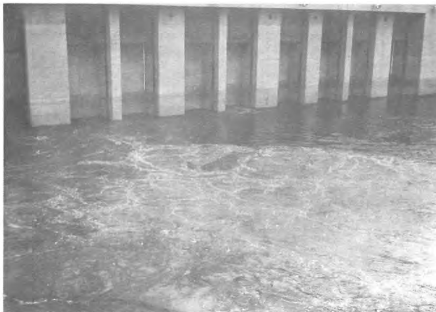
Figure 22. Flatiron Power and Pumping Plant--Flow Conditions in Tailrace Downstream of By-Pass Valve Stilling Basin--Valve Fully Open.
