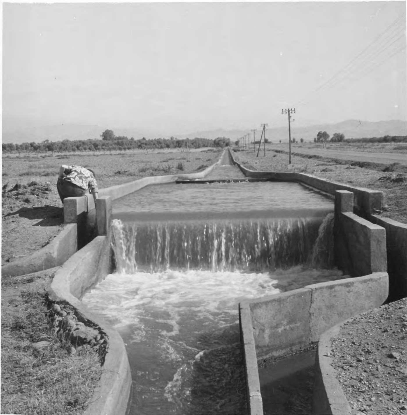
Figure 7. Divisor in Old Irrigation System in Morroco
