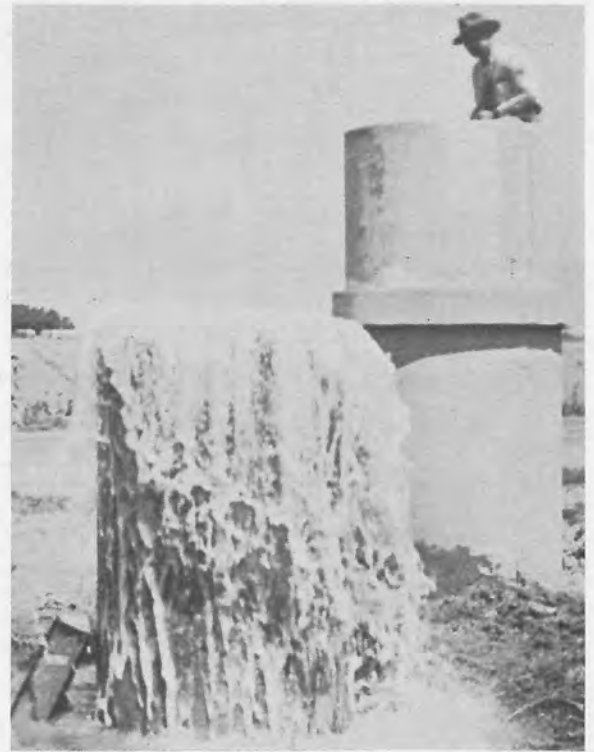
Fig. 2—Surges in pipe stand cause meter stand to overflow
