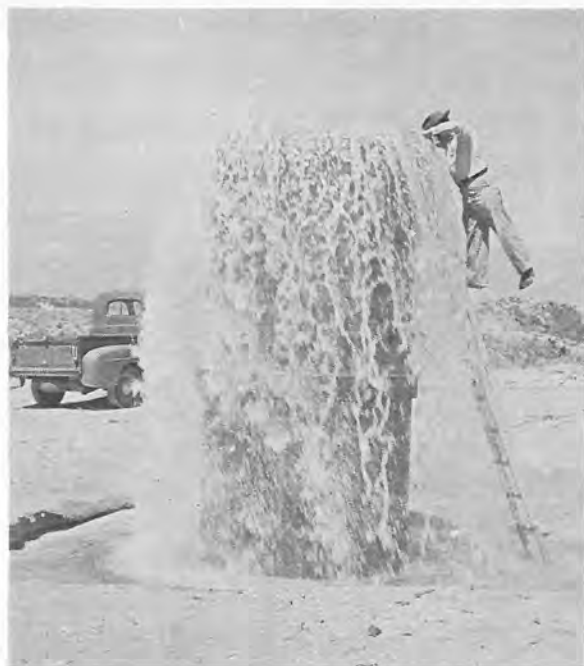
Fig. 1—Pipe stand overflowing due to line surge
