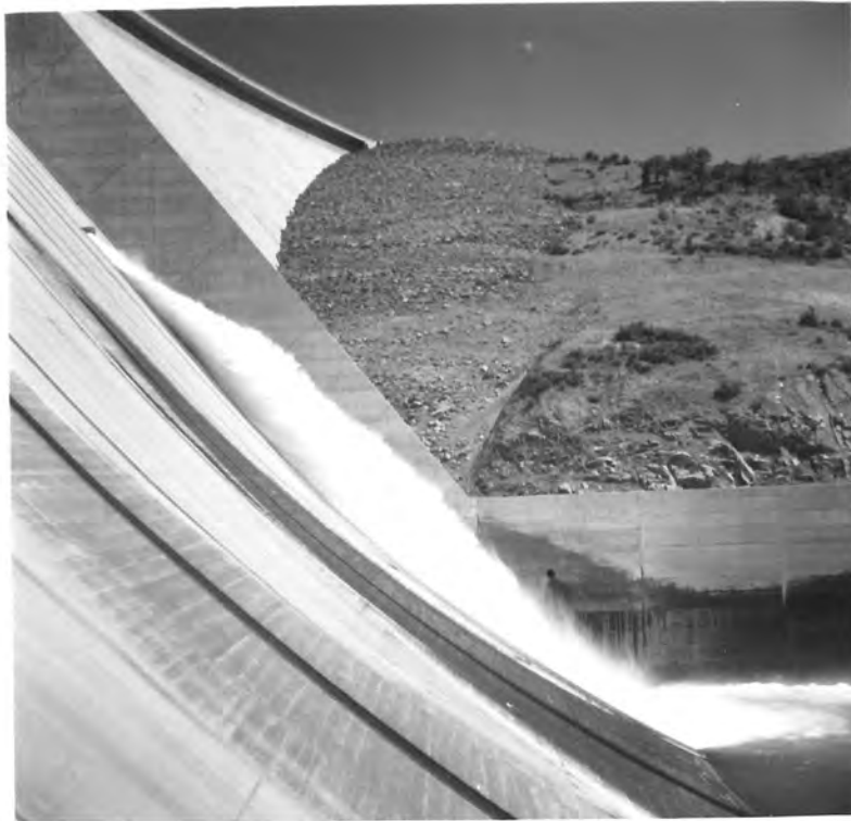
A - Outlet 1 discharging at a small opening.
