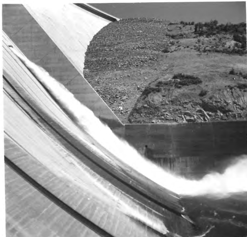
B - Outlet 1 discharging at the wide open position.
