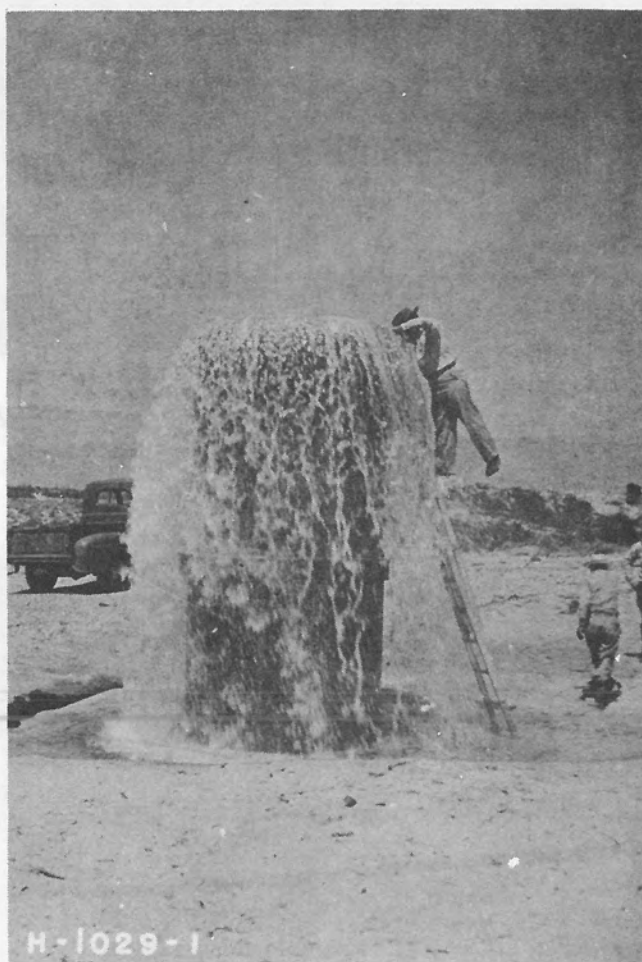
Figure 22c. Surges in pipe line distribution system cause overflow at weir stand.
