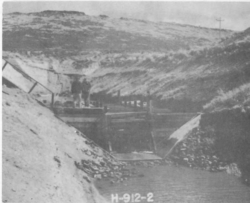
Figure 25. A typical weir installation for the measurement of discharge for pump efficiency test.
