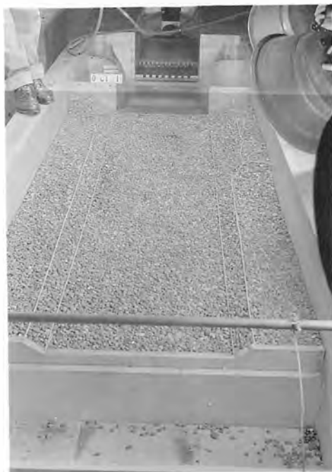
C. PARSHALL FLUME LOOKING UPSTREAM
