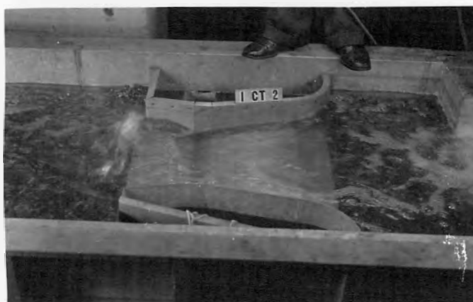
C. PARSHALL FLUME ORIGINAL DESIGN
