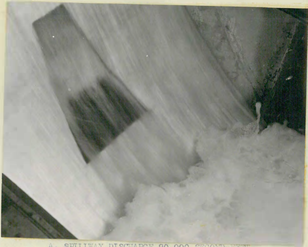
A. SPILLWAY DISCHARGE 90,000 SECOND-FOOT 10 FLO I OUTLET. AIR VENT OPEN.
