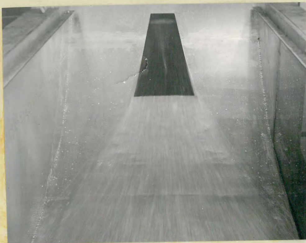
A. OUTLET DISCHARGE 4,700 SECOND-FOOT HEAD= 190 FEET ON ELEV. 358.00
