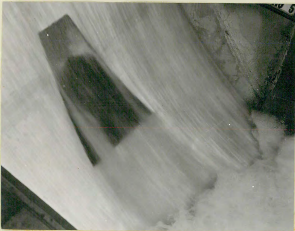
B. SPILLWAY DISCHARGE 90,000 SECOND-FOOT OUTLET DISCHARGE 4,700 SECOND-FOOT HEAD= 190 FEET ON OUTLET (60 FEET 35.00)
