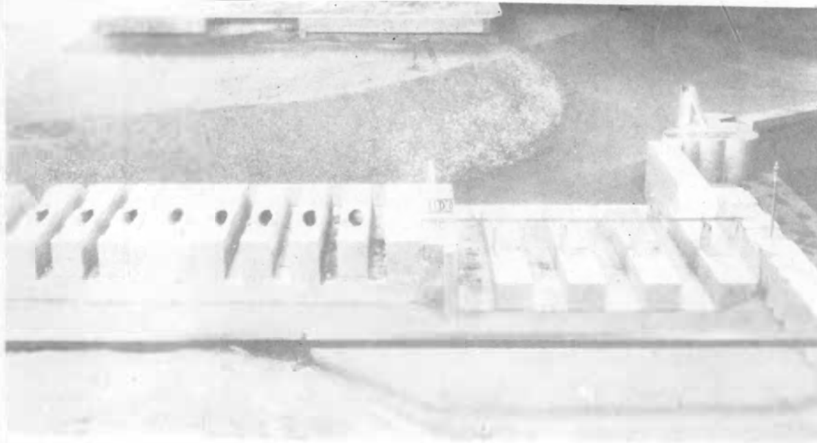
Upstream Side of Dam.
