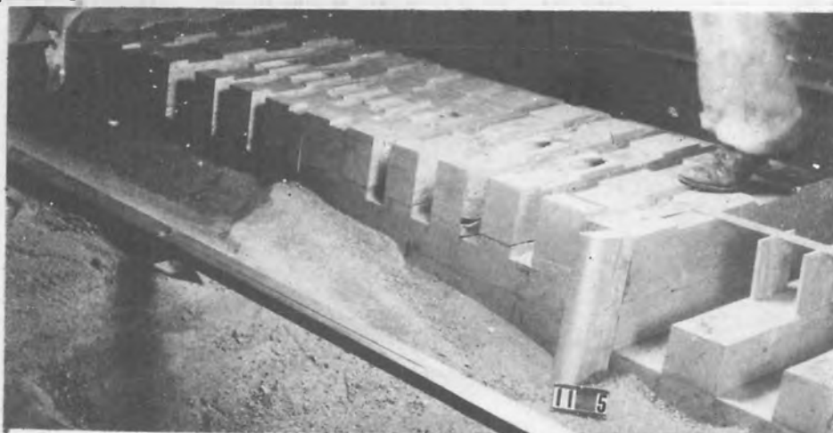
Upstream Side of Dam.
