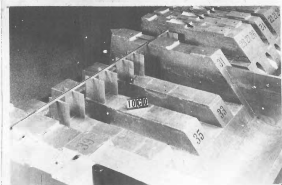
Close up of Spillway Section Showing Trestle Bents.
