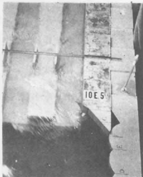
Wooden Crib at Upstream End of Block 39 - Discharge 500,000 Second-feet.
