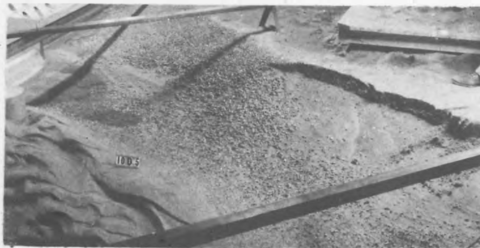
Left Bank below Riprap and River Channel below Dam.
