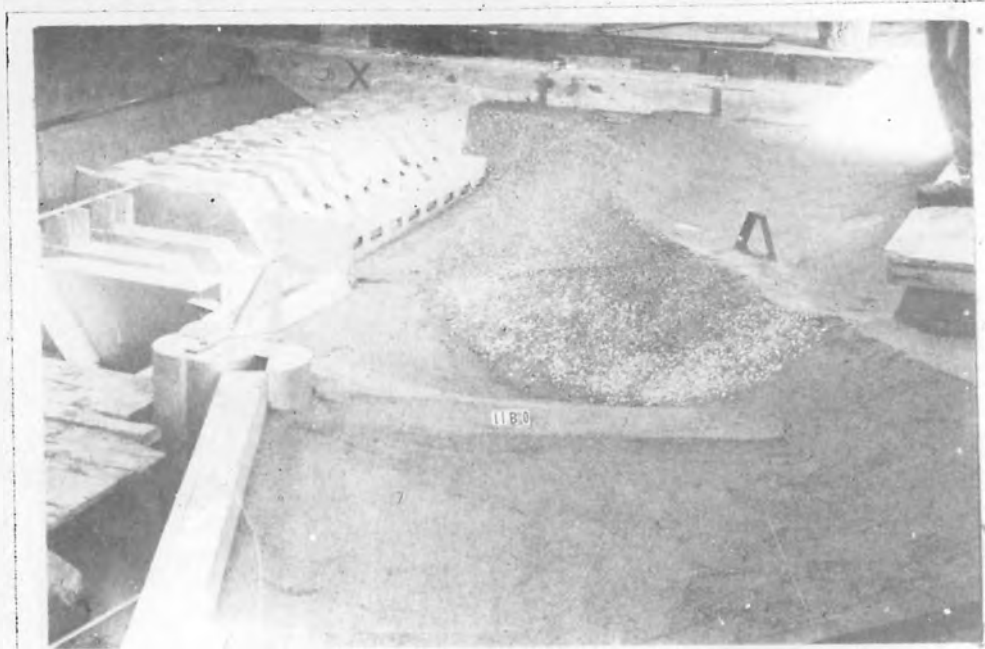
Looking Upstream from Right Bank.
