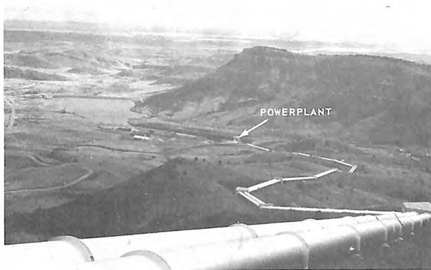
Flatiron Powerplant Penstocks—Butterfly Valve House Behind Camera—Radioisotope Discharge Measurement Section in Foreground on Right Hand Penstock. Photo P245-D-60413NA
