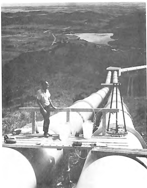
Sampling Equipment Installed at Manway for Integrated Sample and Dilution Methods of Measurement. Photo P245-D-63688NA
