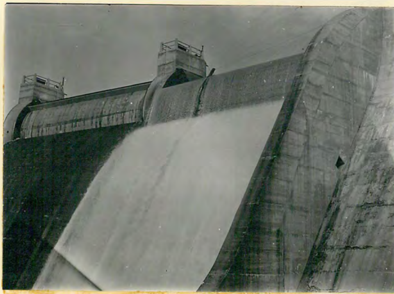
LOG ON ONE-THIRD POINT ON NO. 1 GATE SHOWING FLUTTER OF TWO-THIRDS PORTION OF JET HEAD ON GATE 0.4 FT.
