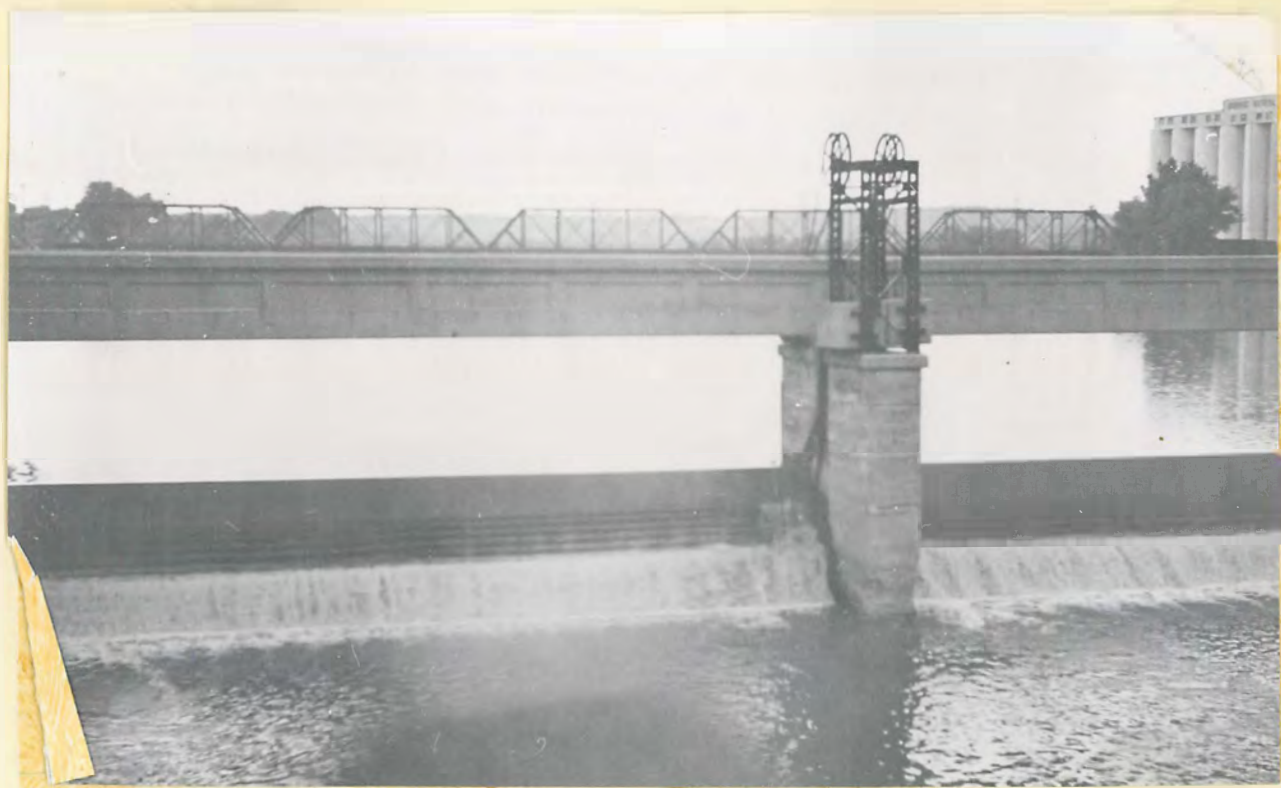
VIBRATION OF JET FROM WEIRS ON DAM IN CEDAR RIVER, CEDAR RAPIDS, IOWA
