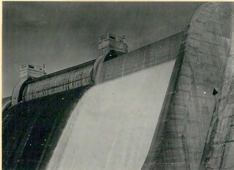
FLUTTER OF JET ON NO. 1 GATE BEFORE LOG WAS PUT IN PLACE HEAD ON GATE 0.4 FT.
