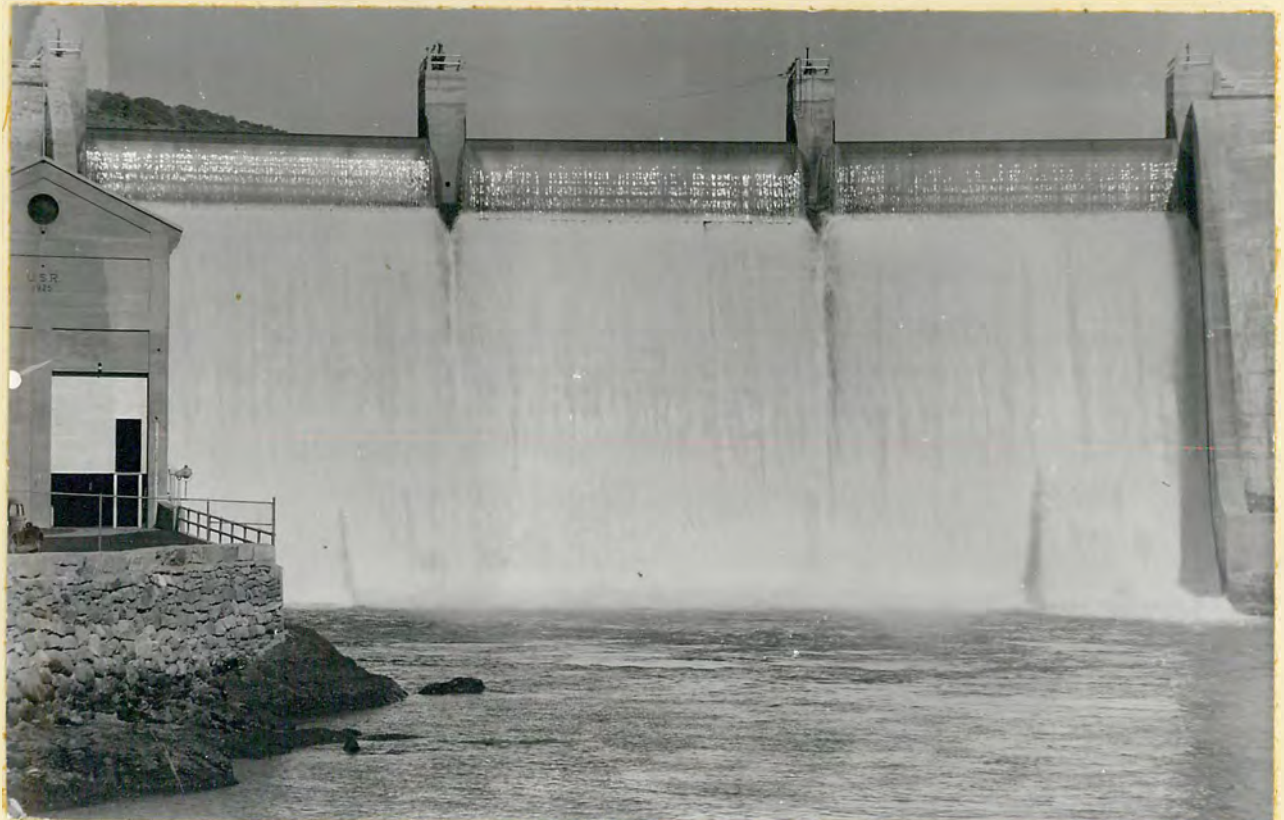
OSCILLATION OF JETS FROM ALL THREE GATES - GATES RAISED 7.6 FEET - HEAD ON GATES 1.15 FEET
