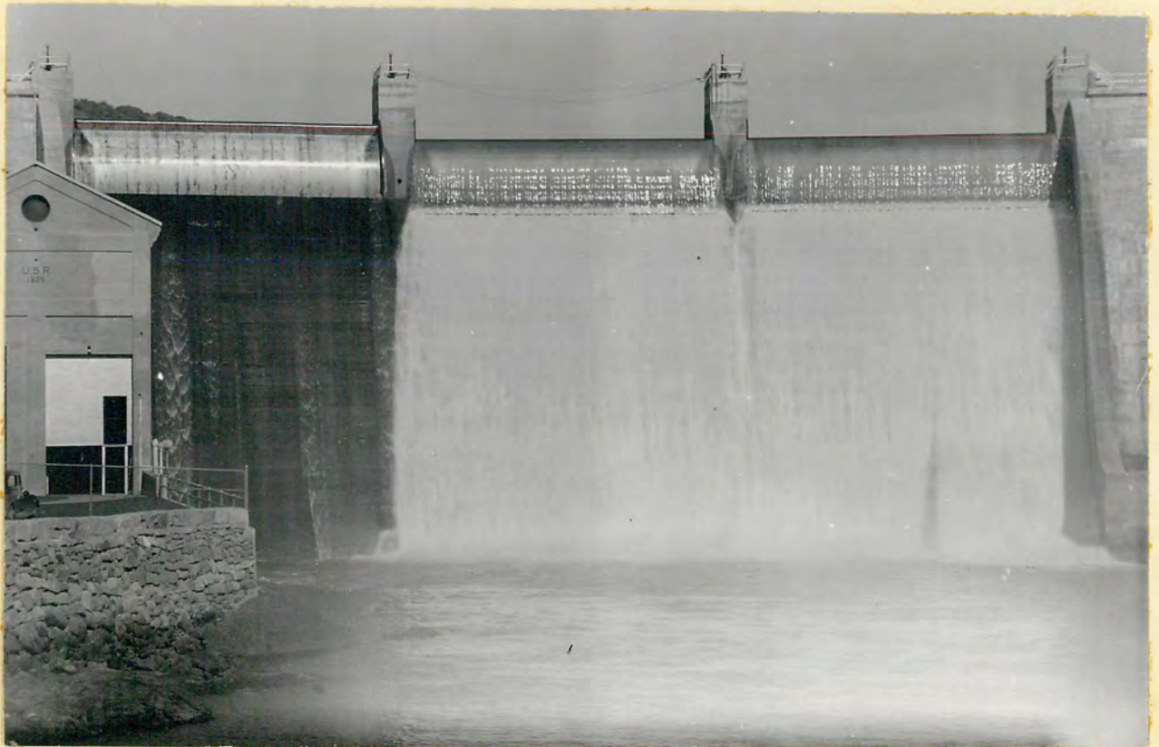
OSCILLATION OF JETS FROM NO. 1 AND NO. 2 GATES - GATES RAISED 7.6 FEET - HEAD ON GATES 1.15 FEET
