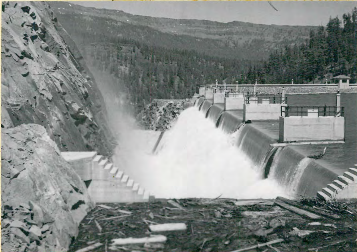
65- BY 8-FOOT DRUM GATES ON TIETON DAM SPILLWAY GATES COMPLETELY RAISED - SMALL HEAD OVER GATES
