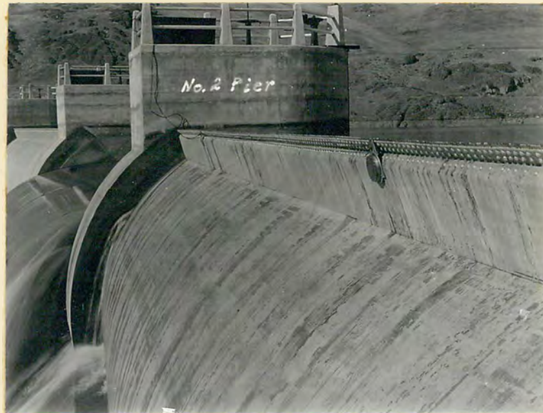
PRESSURE CELLS ON LIP OF NO. 1 GATE CARBON PILE PRESSURE CELL - LEFT MOVING-COIL PRESSURE CELL - RIGHT
