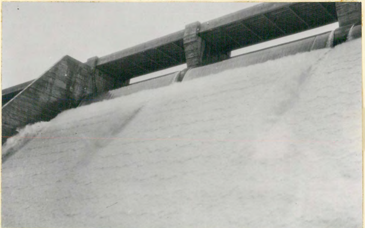
DISCHARGE OF 2,000 SECOND-FEET OVER NORRIS DAM SPILLWAY RESERVOIR ELEVATION 1030.4 - GATE CREST ELEVATION 1028.7 FIXED SPILLWAY CREST ELEVATION 1020
