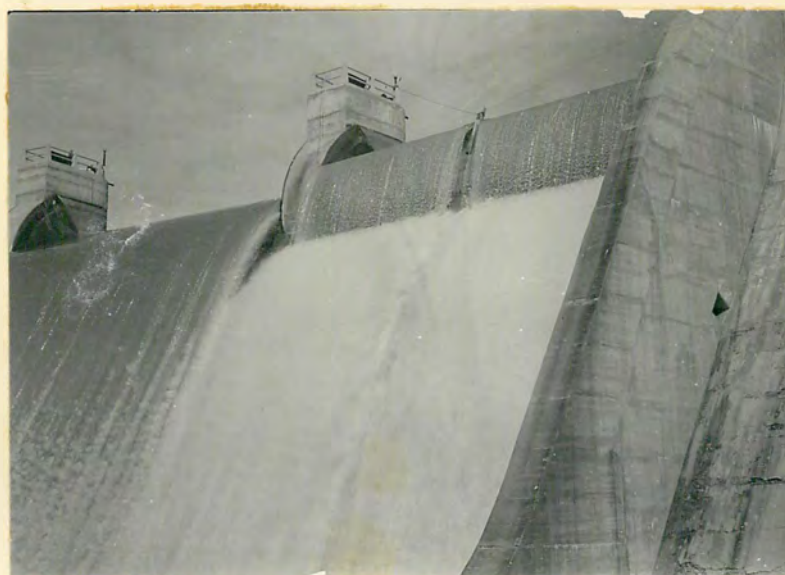
LOG AT CENTER OF NO. 1 GATE - FLUTTER CEASED HEAD ON GATE 0.4 FT.
