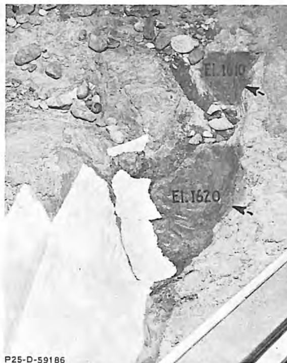
A. First and second ridges are removed to the elevation shown. Ridge locations are indicated by the arrows.
