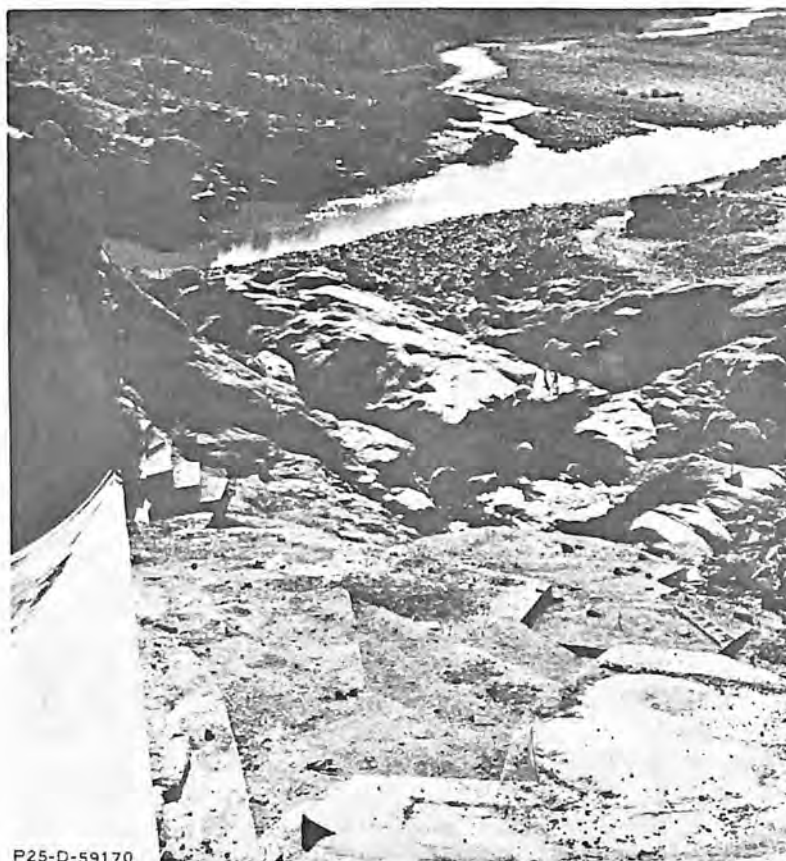
BARTLETT DAM SPILLWAY DISCHARGE CHANNEL EROSION AND REPAIRS PRIOR TO THE 1965-66 FLOOD
