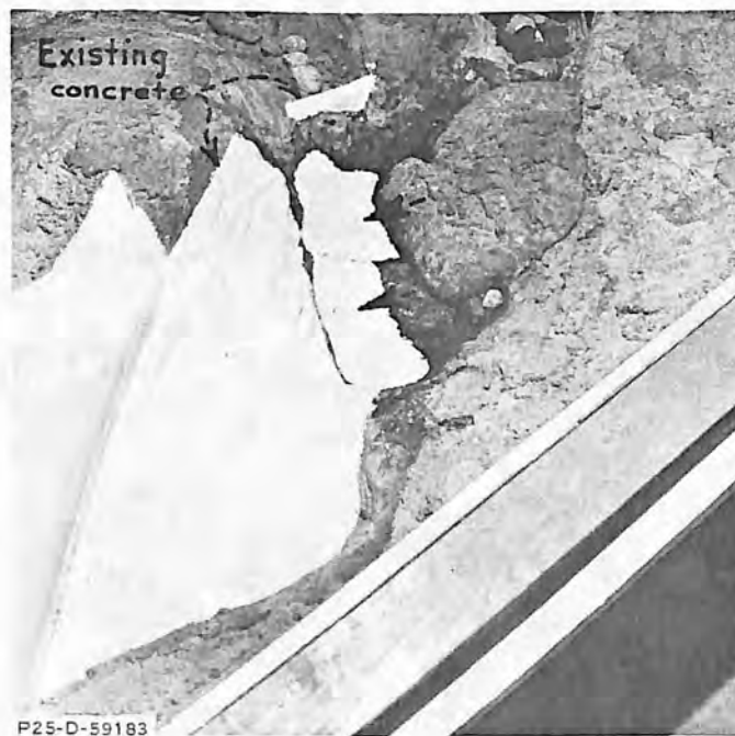
B. Recommended additional concrete fill is indicated by the arrow
