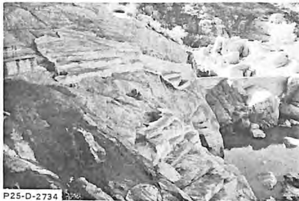
A. Note the undermining of previous channel repairs.
