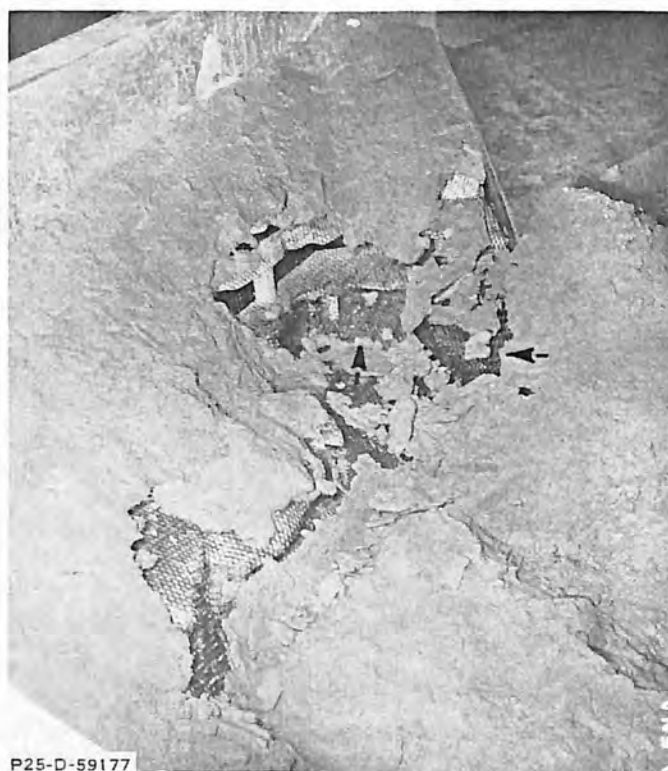
C. Erosion resulting from flows of 30,000 and 175,000 cfs (849 and 4,952.5 cms)
