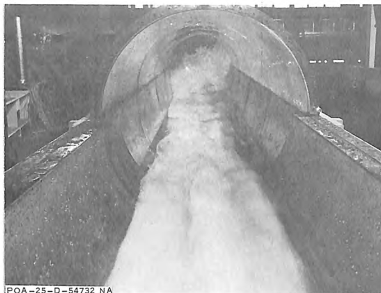
A. Both gates discharging 5,000 cfs Reservoir El. 2100. Looking downstream.
