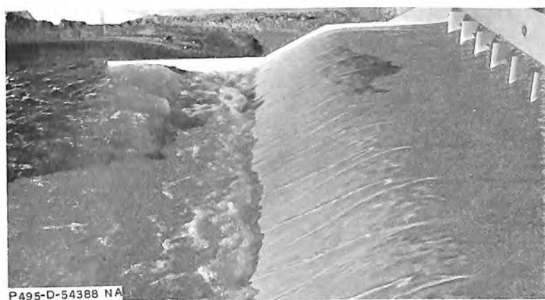
Discharge 264,500 cfs with gates fully open reservoir water surface El. 1492.2
