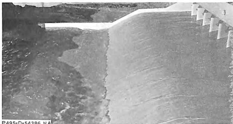
Discharge 132,250 cfs with gates fully open reservoir water surface El. 1482.9
