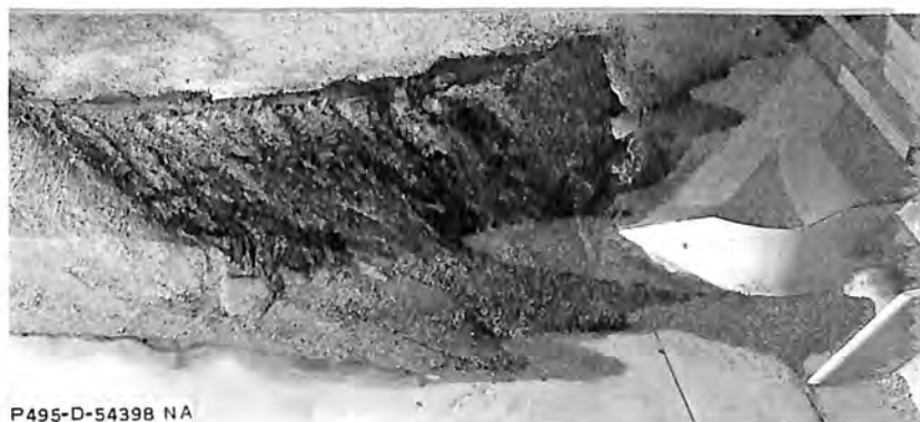
B. The eroded area along the left side slope extended about 350 feet upstream from the spillway crest after operation at the above discharge
