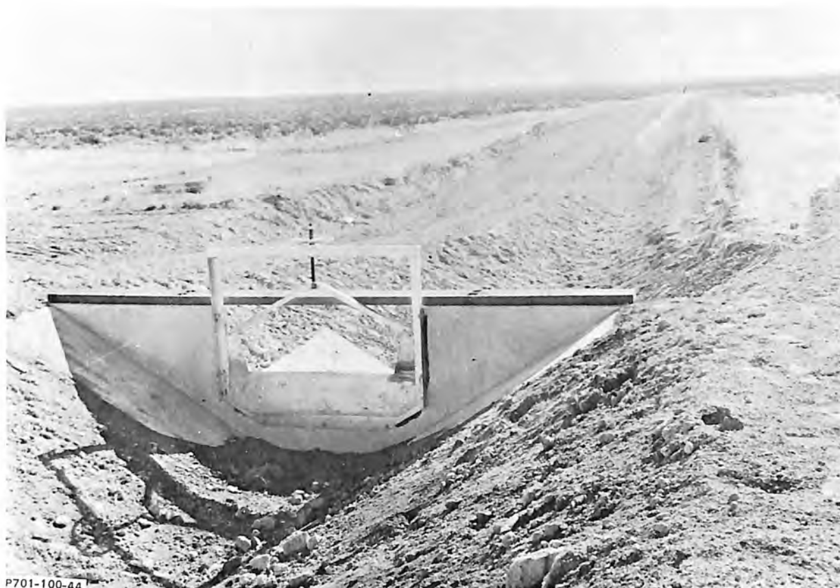
A. Four-foot adjustable weir used as a combination check and measuring structure--North Side Pumping Division Minidoka Project, Idaho
