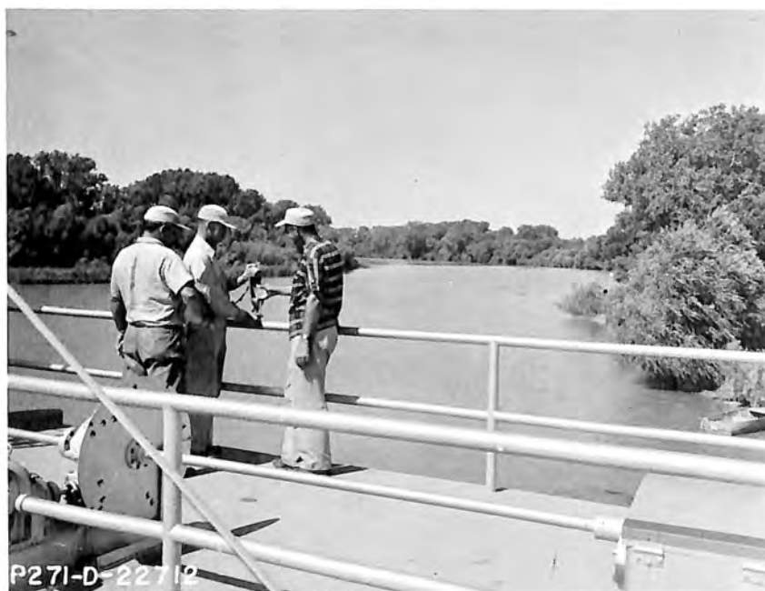
B. Sampling with suspended sediment sampler DH-59 at entrance to sluiceway--Superior Canal head-works.
