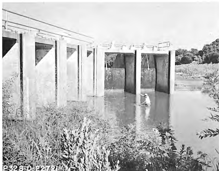
A. Measuring water depth and sediment deposit upstream from headworks and sluiceway.
