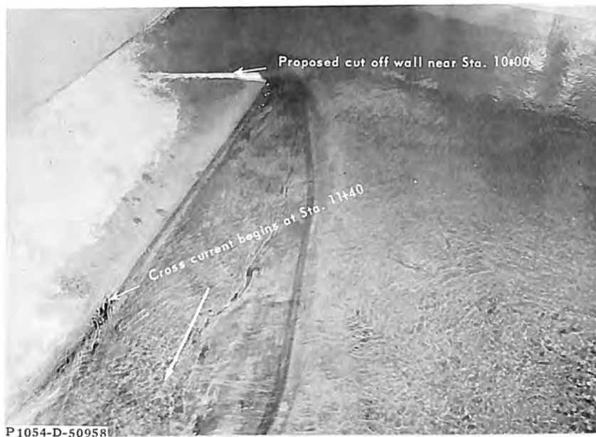
A. Upstream end of spillway.
