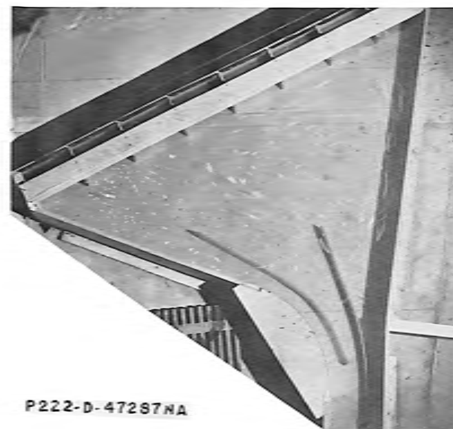
B. Angled transition with curved guide walls.
