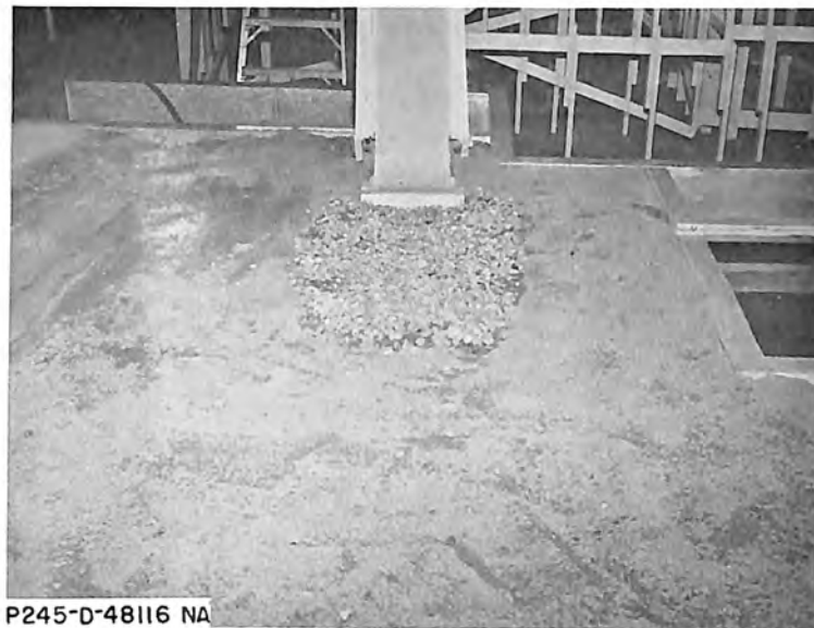
A. Riprap lined channel extending 150 feet downstream from bucket
