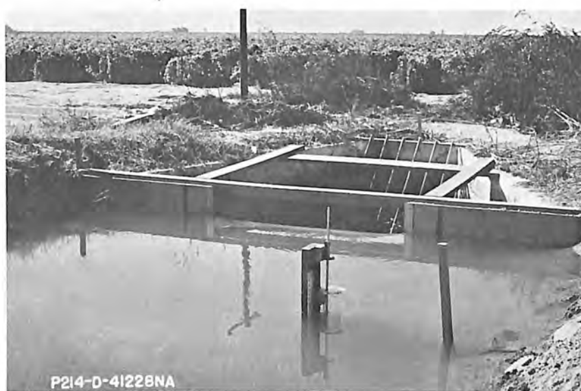
B. Weir performance with discharge of 24.9 cfs.
