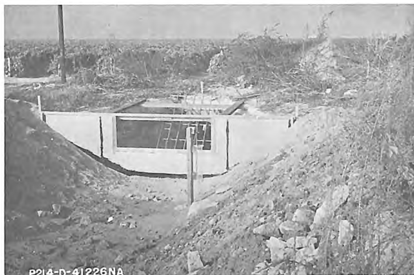
A. Six-foot-long fully contracted rectangular weir and head gage installed at road crossing transition structure, Station 173+80.
