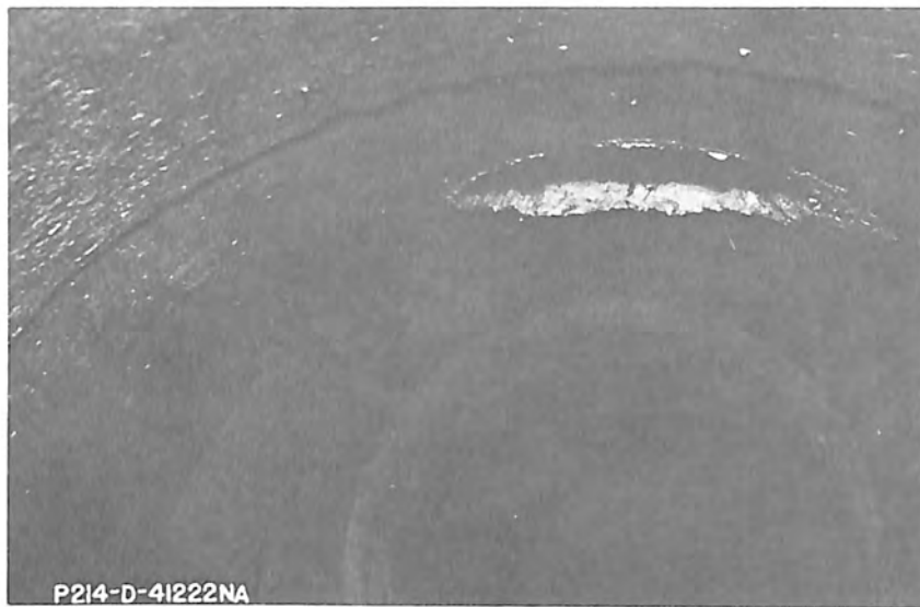
A. Vent in crown (light area) of 42-inch cast-in-place pipe, showing slight mortar protrusions, Station 293+00.
