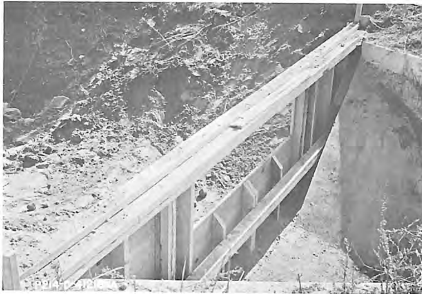
A. Weir frame and bulkhead installed against road crossing transition structure.
