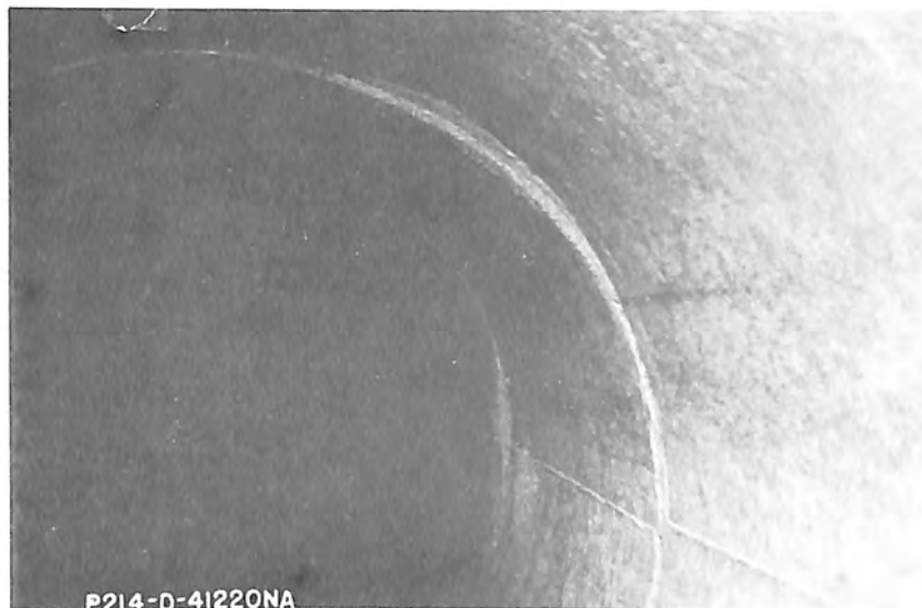
B. Surface of 48-inch cast-in-place pipe showing mortared offsets near Station 260+50, direction of flow is toward the viewer.
