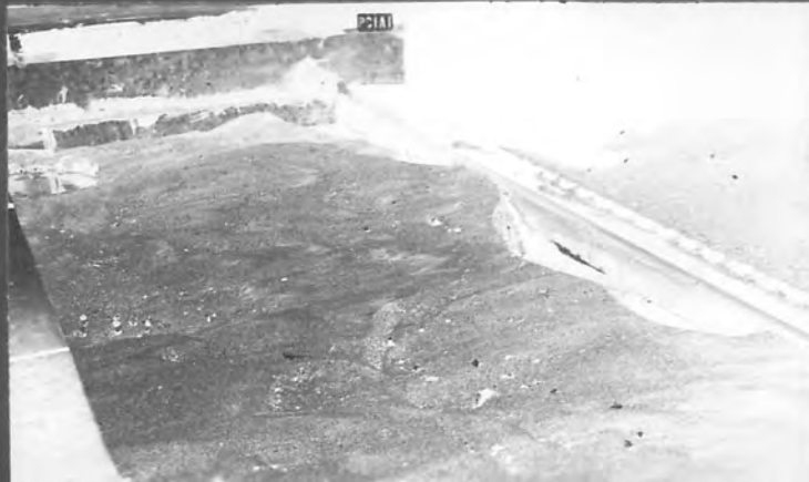
Figure 13 - Holes Scoured Upstream From Crest of Salt River Power Canal Diversion Dam.
