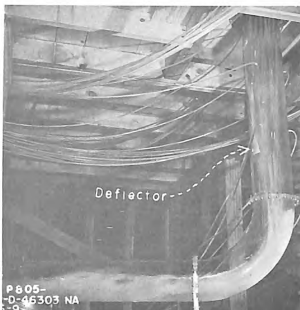
B. Deflector ends at elevation 485 in vertical shaft.
