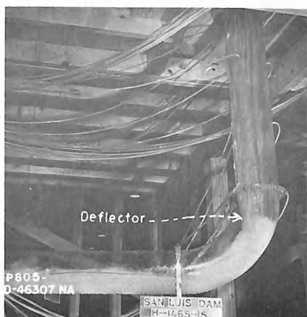
D. Deflector extending into vertical bend.
