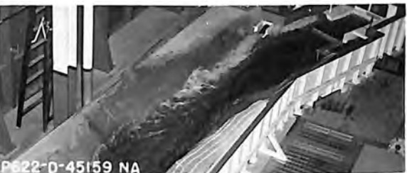
E. Spillway--5,500 cfs Outlet works--5,100 cfs Powerplant--3,080 cfs
