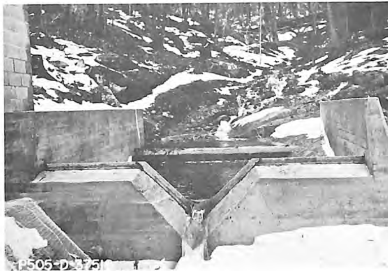
A. Compound weir, 90° V-notch with horizontal extensions, used to measure stream flows by the United States Department of Agriculture Forest Service.
