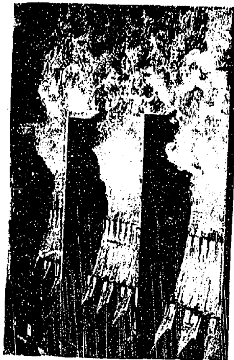
D. DISCHARGE 24,000 SECOND-FeET TAILWATER ELEVATION 150 JUMP ON VERGE OF SLAVING POOL.
