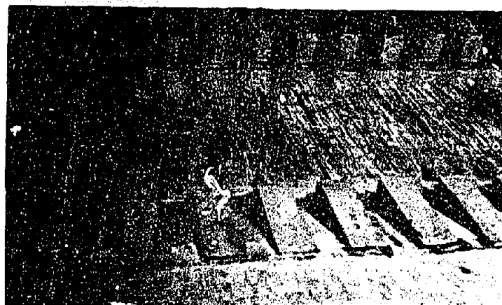
A. STILLING POOL. LOOKING DOWNSTREAM.
