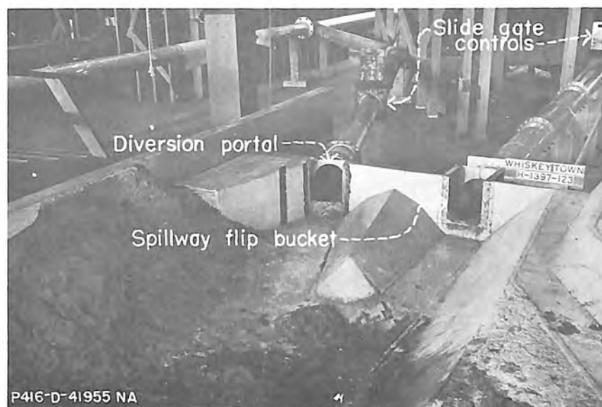
A. Diversion tunnel outlet portal and spillway flip bucket.
