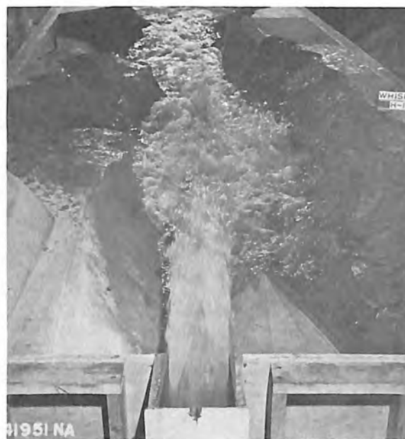
C. 14,250 cfs - Tailwater elevation 965.4
