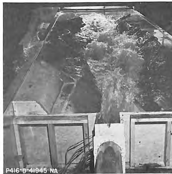
D. 28,780 cfs - Normal tailwater.
