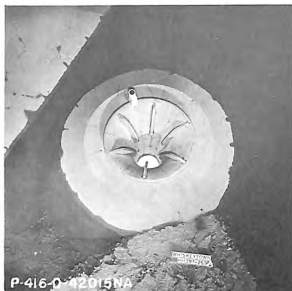
A. Six rib vanes, air vent pier and 4'-8" deflector in bend.
