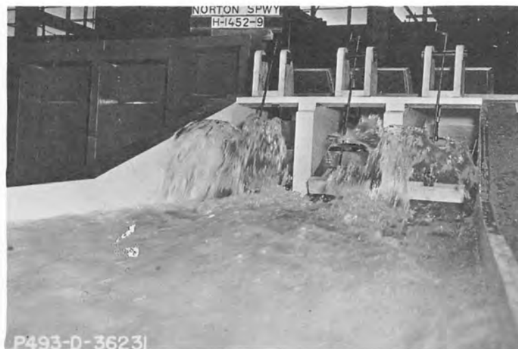
Flow impinging on counterweights.
