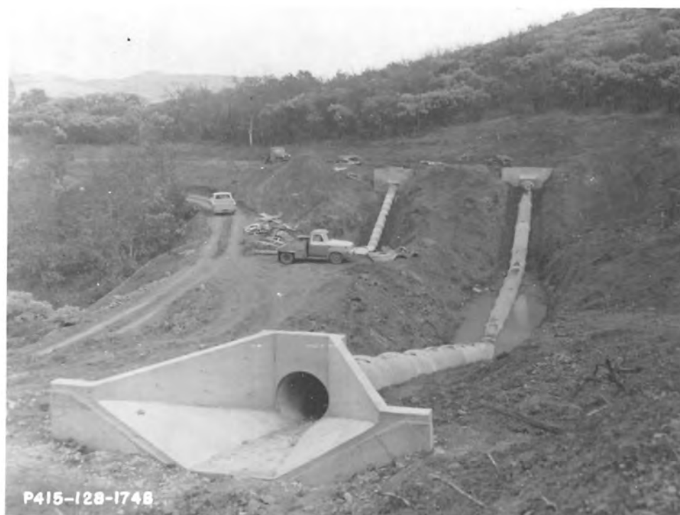
Siphon outlet at Station 521, West Lateral Rogue River Basin Project, Oregon. November 1961.
