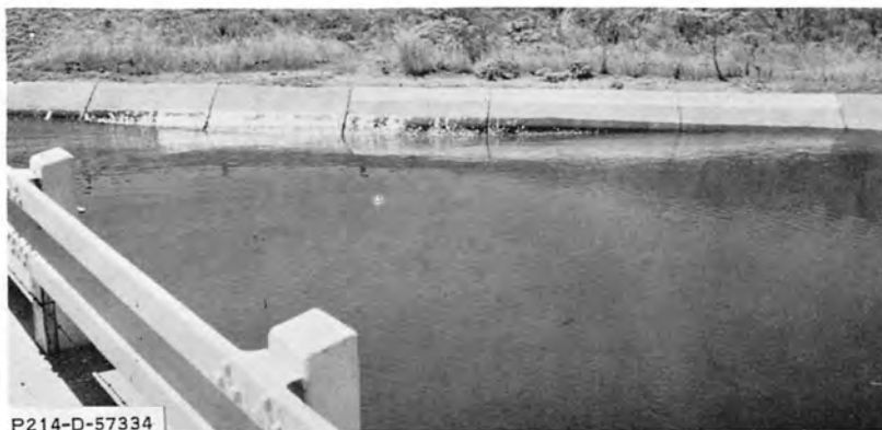
B. Bridge Mile 56.60--Wave formed at upstream right side of canal, Abutment 1, Figure 1.
