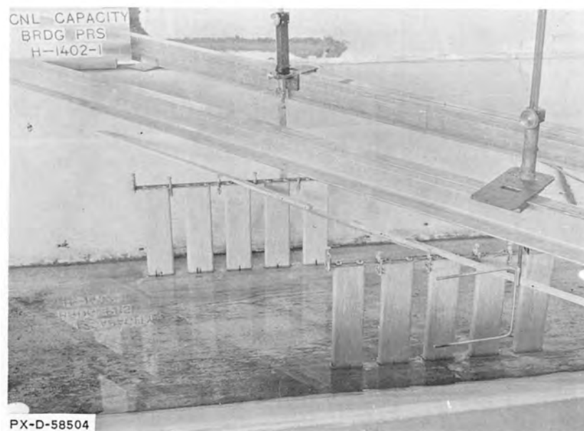
C. Capacitance probes and point gage staff mounts.
