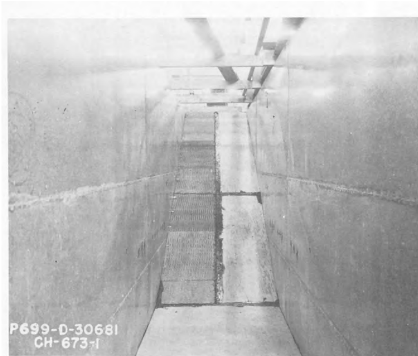
Plywood Support For Simulated Canal Slope And Bottom. Left Half Of Slope Is Covered With Metal Lath Simulating A Rough Subgrade East Bench Canal Drawdown Tests 1:1 Scale Sectional Model
