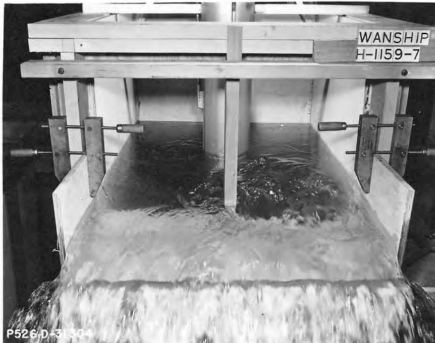
A. Water depth from top of pedestal = 10.2 ft. Note surge on smooth water surface.
