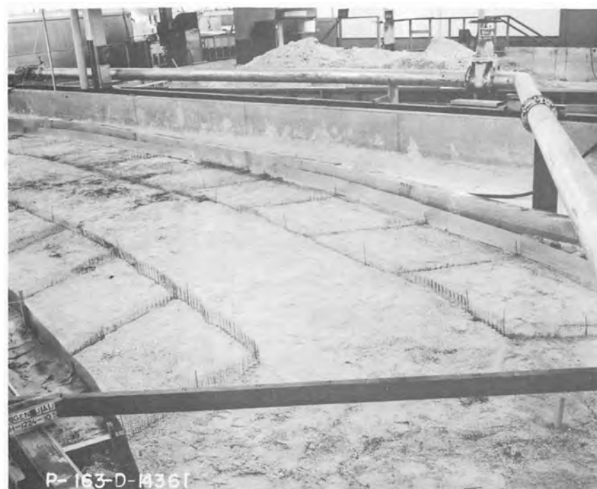
(b) Downstream view
