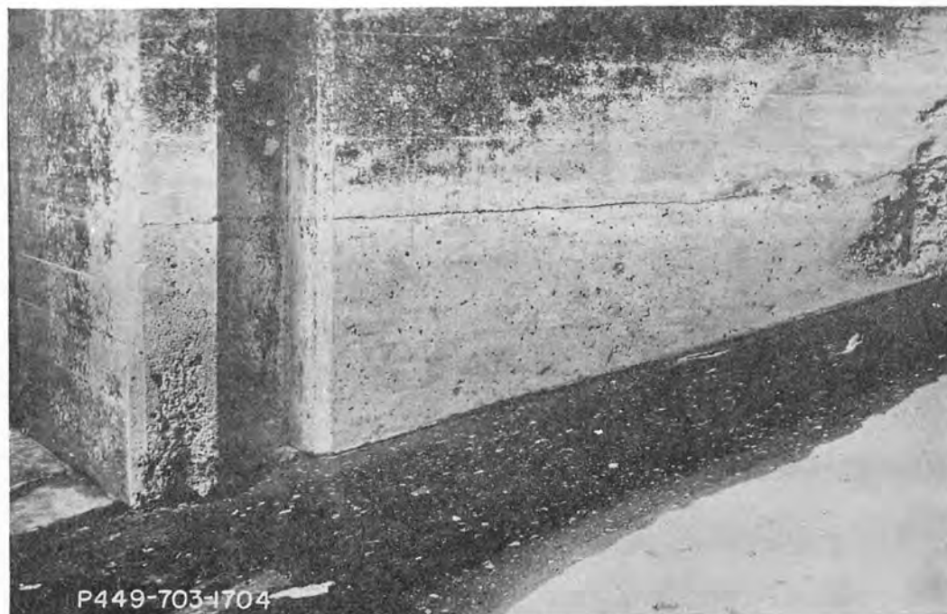
A. Right flared wall of Outlet Bay 3. Maximum depth of erosion is 3 inches at flared wall and 8 inches in floor at stop-log slot.
