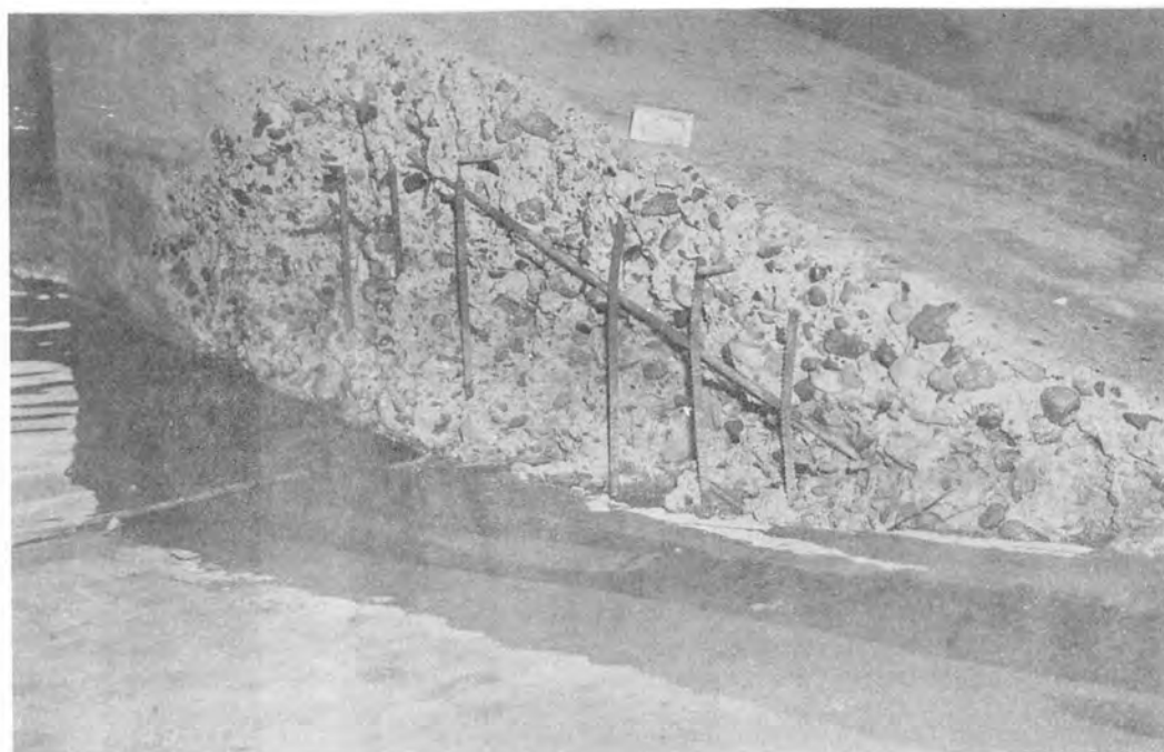
B. Left side of center chute block in Outlet Bay 2. Maximum depth of erosion is 17 inches.
