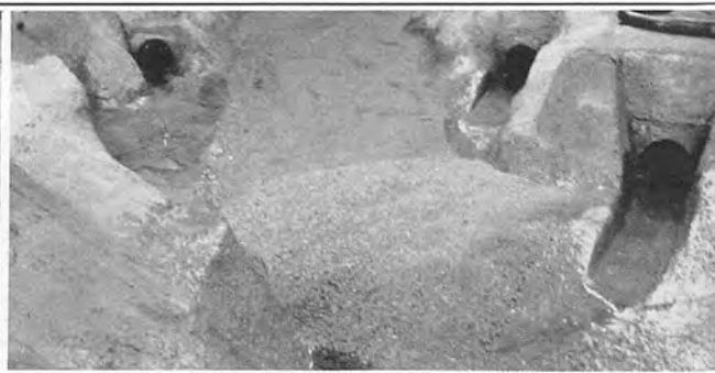
A. Normal Tailwater B. Erosion of River Bed Always 200,000 Second-Feet, Canyon Wall Outlets 42,000 Second-Feet, Tunnel Plug Outlets 46,000 Second-Feet, Powerhouse 15,000 Second-Feet
