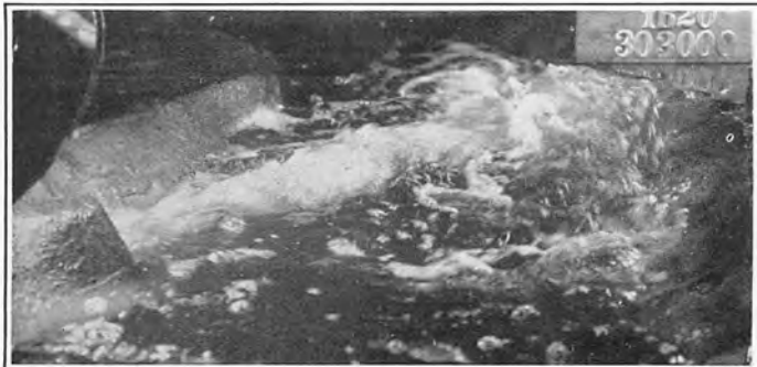
C. Normal Tailwater D. Erosion of River Bed Arizona Spillway 200,000 Second-Feet, Canyon Wall Outlets 42,000 Second-Feet, Tunnel Plug Outlets 46,000 Second-Feet, Powerhouse 15,000 Second-Feet
