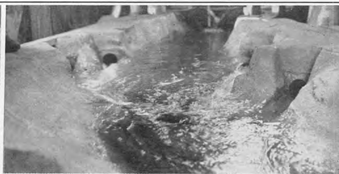
D. Normal Tailwater, Powerhouse 15,000 Second-Feet, Tunnel Plug Outlets 46,000 Second-Feet
