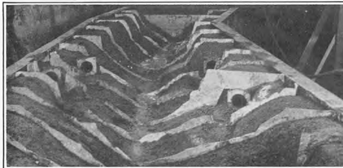
A. Method of Constructing River Bed
