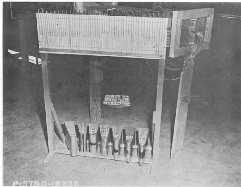
B. Upstream Pier Shape Study Air Model
