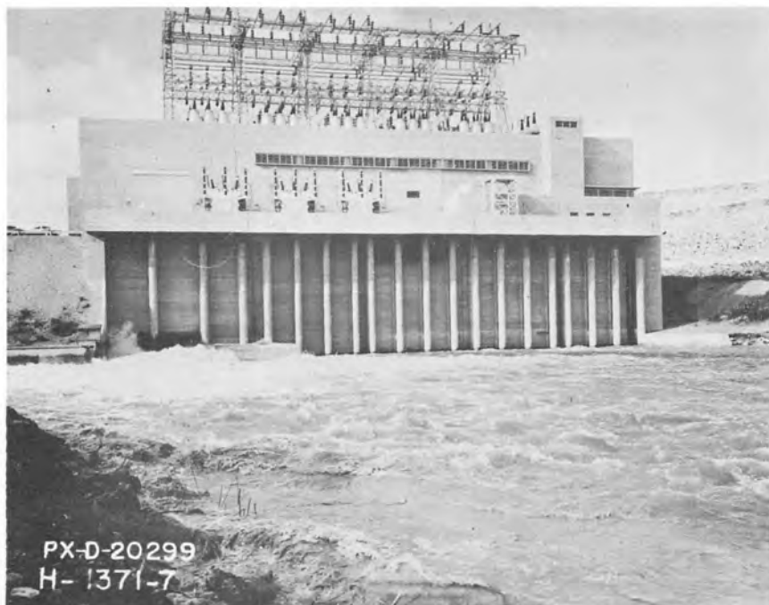
90-inch outlet works valves open 100 percent discharging 4,500 cfs approx. - T. W. elev. 183.6. Turbine gates 72 percent open - 100 percent load.
