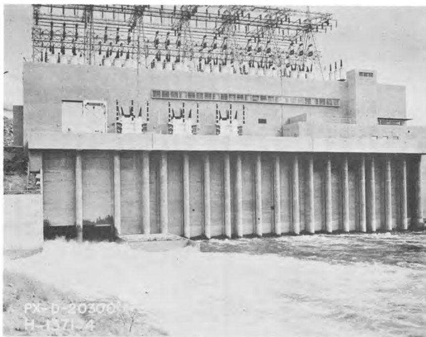
72-inch outlet works valves open 100 percent discharging 3,000 cfs approx. - T. W. elev. 184.1. Turbine gates 72 percent open - 100 percent load.
