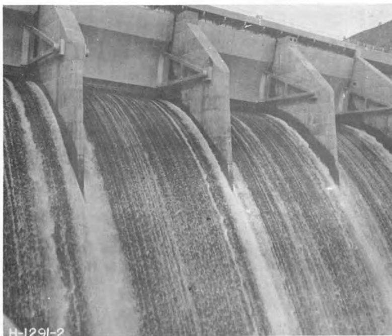
A. Flow Conditions for Discharge of 24,000 cfs with Four Gates Open 4.2 Feet
