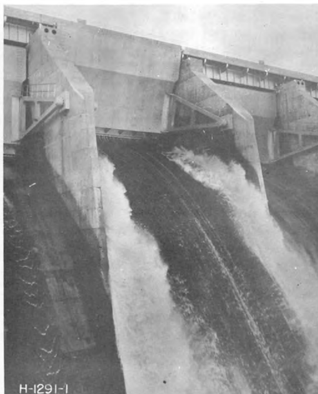
B. Flow Conditions for Discharge of 13,800 cfs--Gate Number 2, 10 Feet Open
