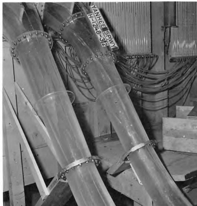
B. Center pier in left tunnel shortened 2 meters. Note increase in height of fin.
