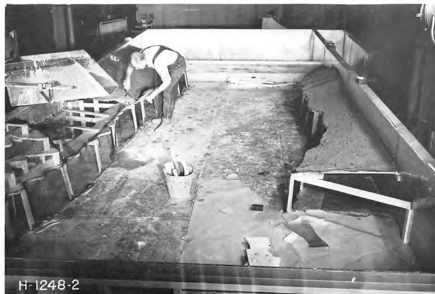
A. Placing topography in tail box.
