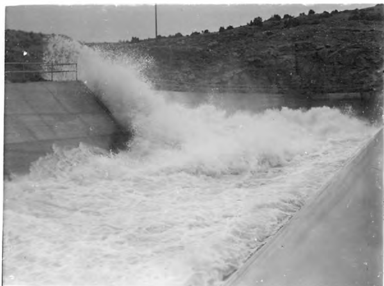
VALVES 100% OPEN - DISCHARGE 4825 SECOND-FEET.
