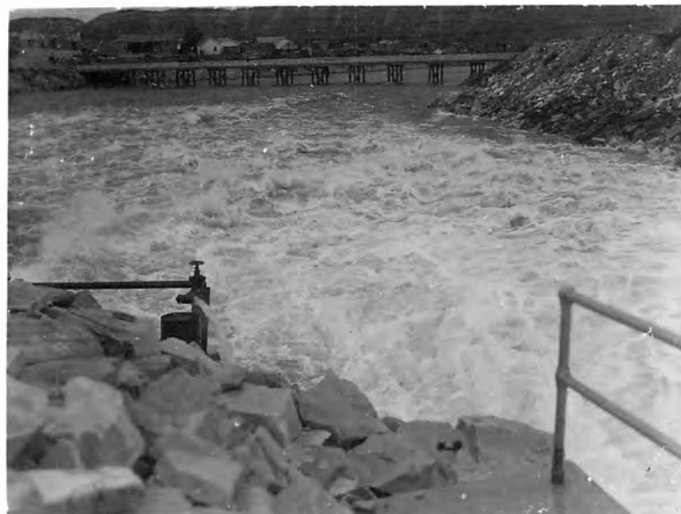
VALVES 100% OPEN - DISCHARGE 4825 SECOND-FEET.
