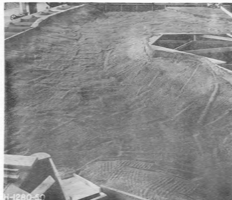
(C) Sand movement in upstream channel following test in (B)
