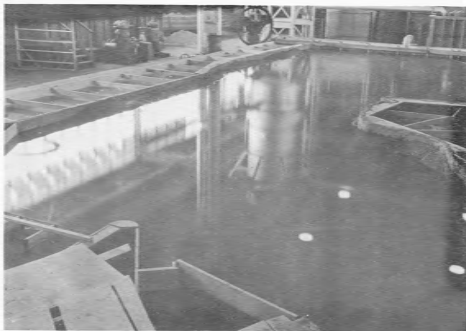
(B) Upstream approach channel flow conditions, discharge representing 5065 cfs, W. S. Elev. +6.0
