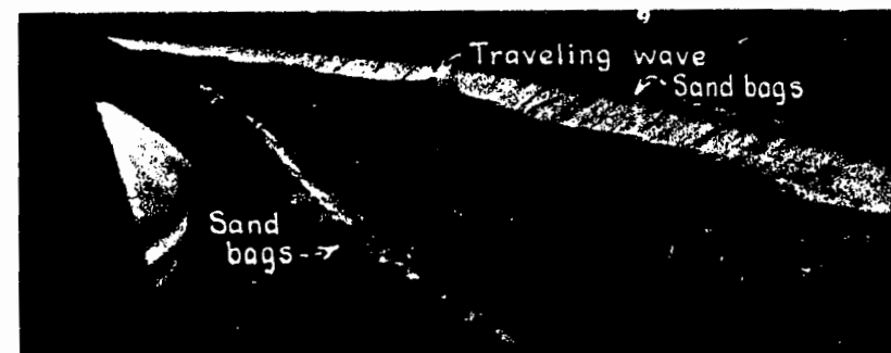
Looking downstream. Waves traveling through the canal over top the canal lining at the horizontal bends.
