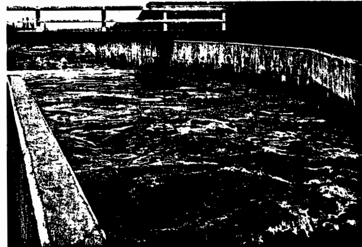
Waves travel through the Parshall flume
