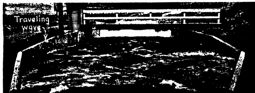
Looking downstream. Waves from the stilling basin travel through the Parshall flume.
