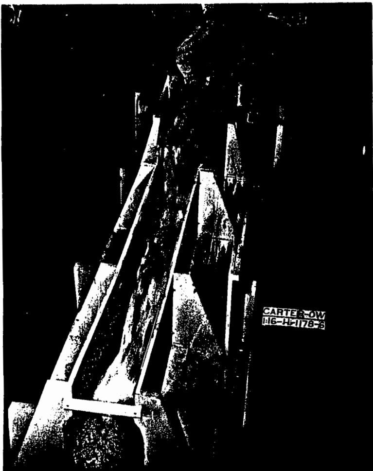
Looking downstream outlet stilling basin and Parshall flume
