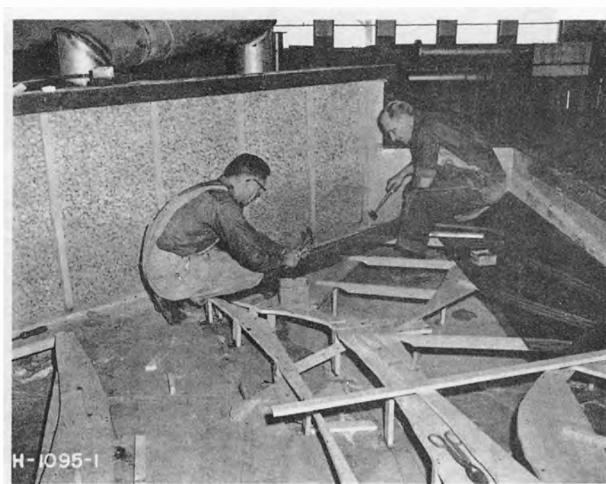
B. Note wood contours being covered with metal lath
